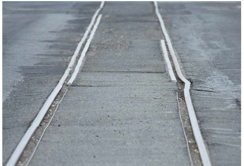
THE YVT TRACK IN THE MIDDLE OF 6TH AVENUE HAS NOT BEEN REBUILT SINCE 1956 AND IT IS SHOWING ITS AGE.
