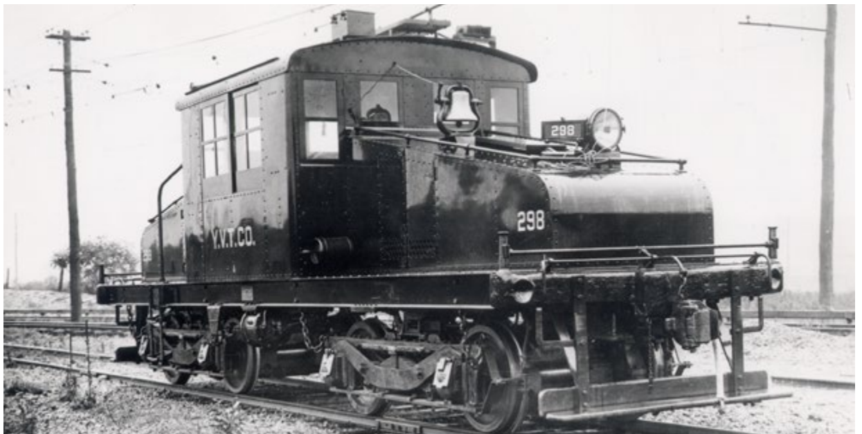
BUILDER'S PHOTO OF STEEPLE CAB #298 WHEN IT WAS NEW FROM GENERAL ELECTRIC
